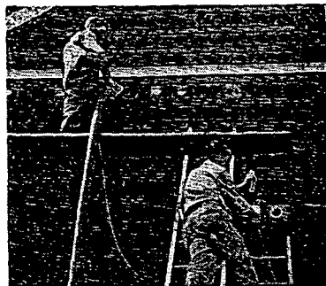
Barrett Rock Wool easily blown through hose into wall and roof spaces. Inside of building not disturbed during application, no opening marks left.
