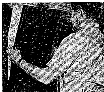
Barrett VB* Batts are imprinted "Barrett." Paper firmly anchored to wool, extends beyond all edges of batt for effective vapor barrier—easy application.
