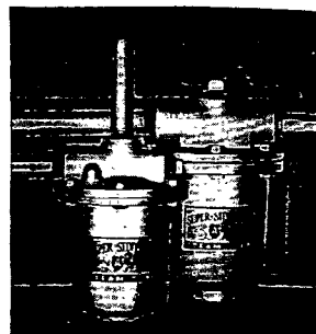
Shows how trap is installed either as an elbow or straight in-line.
