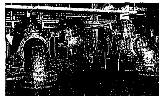
TWO HORIZONTAL SINGLE-STAGE centrifugal pumps develop 37-ft total head to pass 20,500 gpm water through 42,500 sq ft, 2-pass condenser, reversing valves
