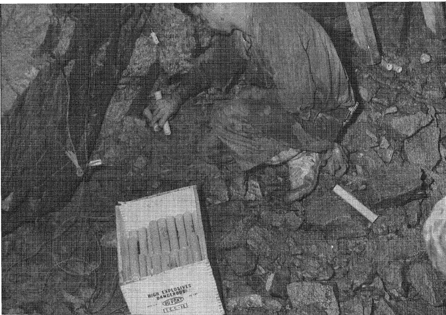
An ore miner prepares a "shot," using Du Pont Series B Delay Electric Blasting Caps.
