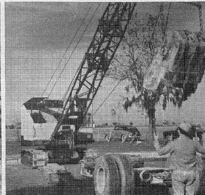
• Loading dragline on the trailer. Nylon truck tires easily take punishing loads like this.
