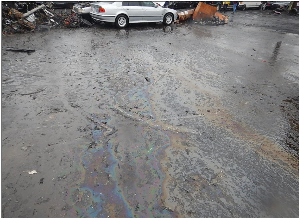
DSCN3886. View, facing west of petroleum sheen west of the crusher. Runoff from this area was flowing toward the southwest perimeter.
