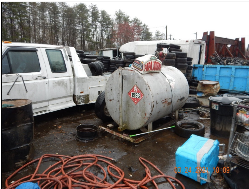
DSCN2131. View, facing south, of an approximately 275-gallon tank located in the southeastern area of the Facility. Note a lack of secondary confinement. It is unclear if there was any liquid in the tank.
