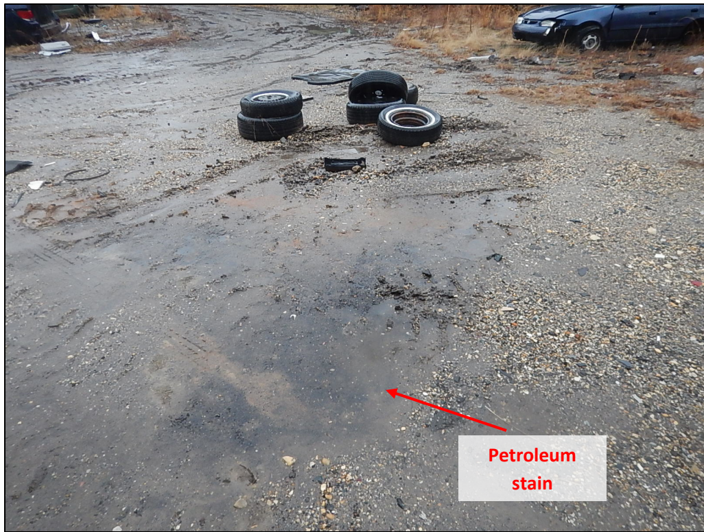
DSCN3786. View of a petroleum stain in the western portion of the Facility.
