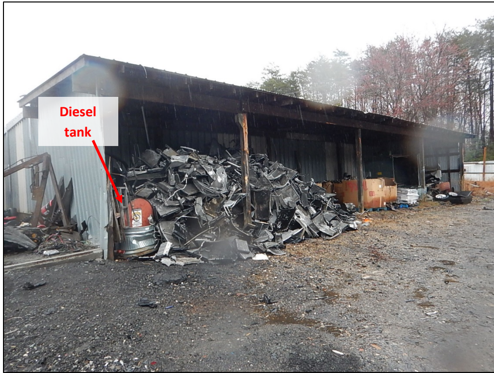
DSCN3904. View, facing east, of the cores/small parts storage area located at the Facility's southeastern perimeter. Note the 275-gallon diesel storage tank underneath radiators. The containment structure was dented.
