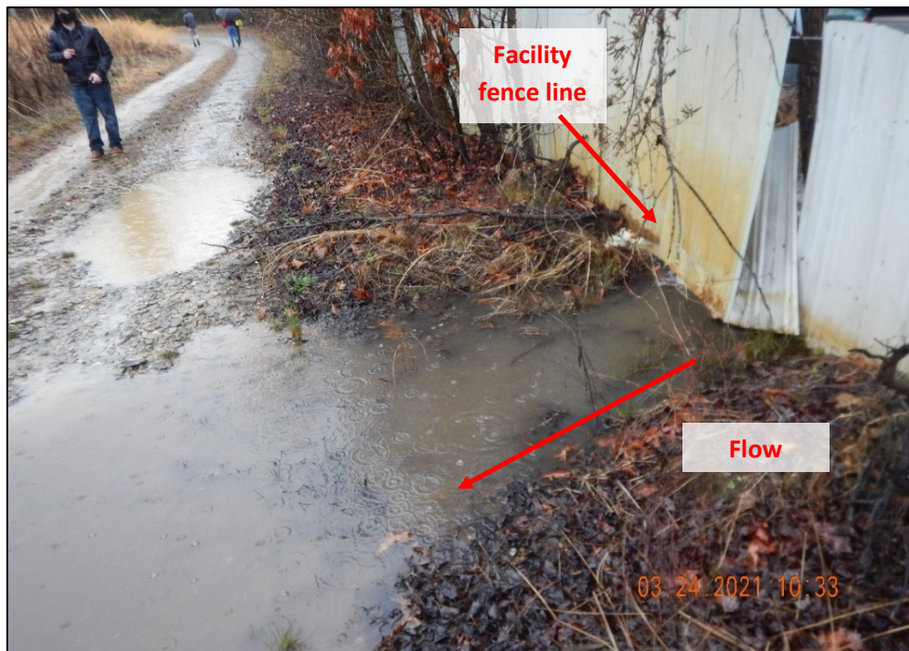
DSCN2169. View, facing west, of runoff leaving the site from the southwest perimeter of the Facility.
