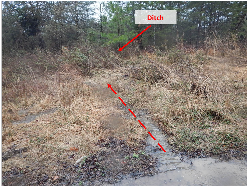
DSCN3971. View, facing southwest, of runoff discharging west of the Facility to the drainage ditch in between the Facility and Huntington Lane.
