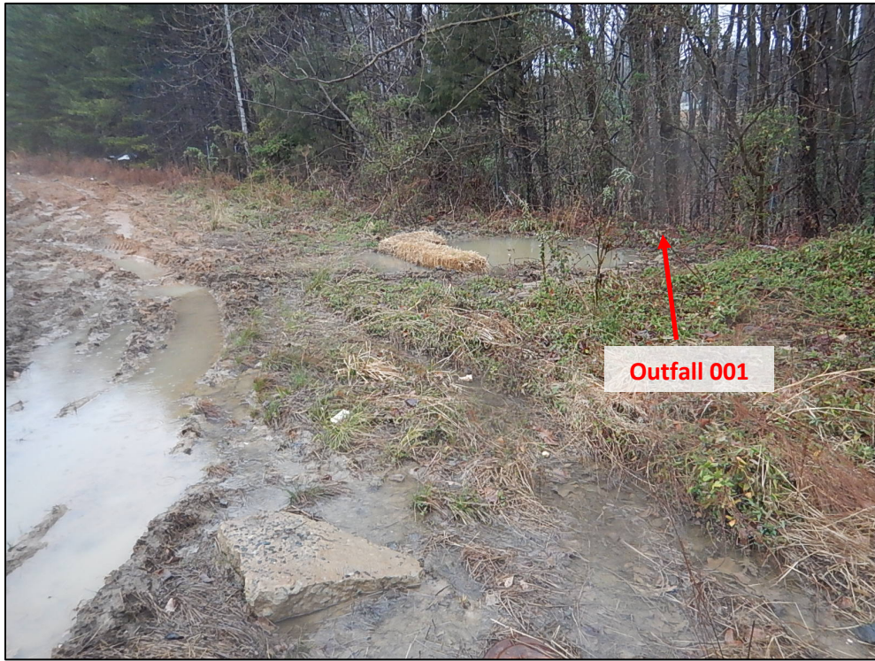
DSCN3749. View, facing northwest, of the ponding area used to collect samples for Outfall 001. Note the area upgradient of the outfall was scoured and muddy.
