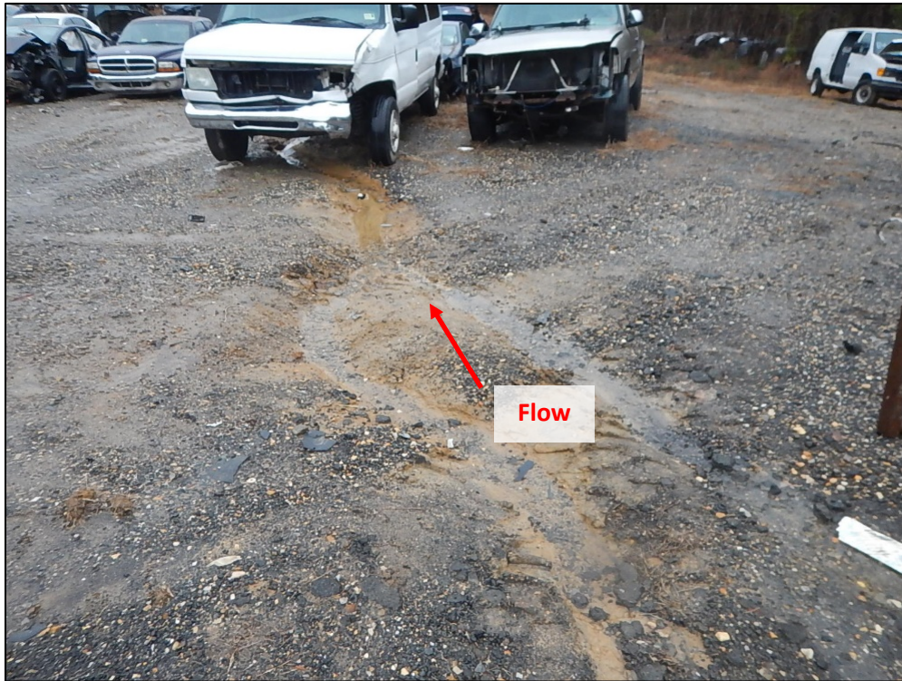
DSCN3737. View, facing northwest, of erosion observed in the lot upgradient of Outfall 001.
