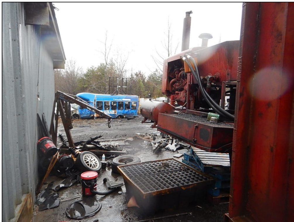
DSCN3919. View, facing south, of the crusher and the pad below it.
