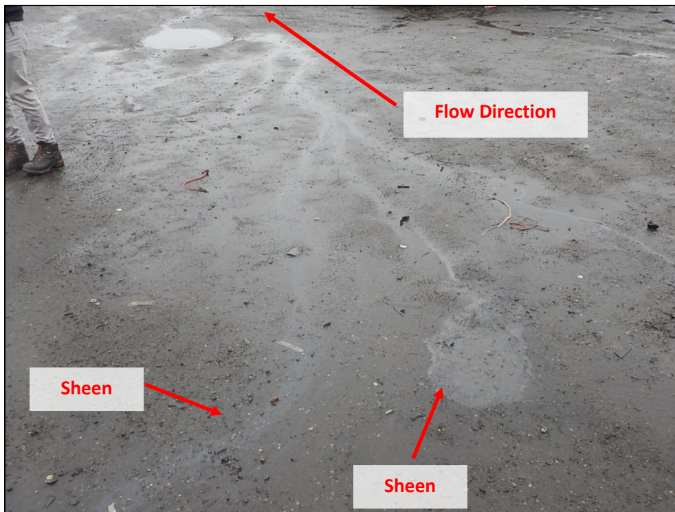
DSCN3713. View, facing west, outside of the dismantling garage. Note the petroleum sheen and flow path of the runoff.
