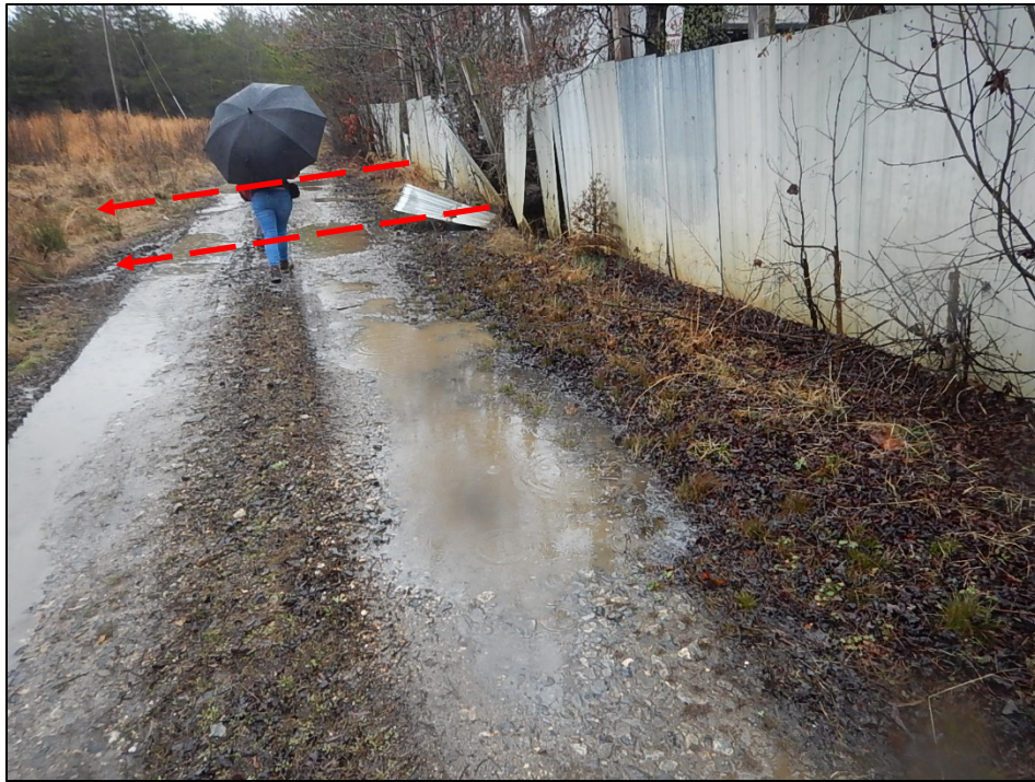
DSCN3960. View, facing northwest, of the southwestern perimeter of the Facility (photograph taken offsite). Note runoff leaving the site in multiple locations. View is immediately northwest of area shown in DSCN3944 .
