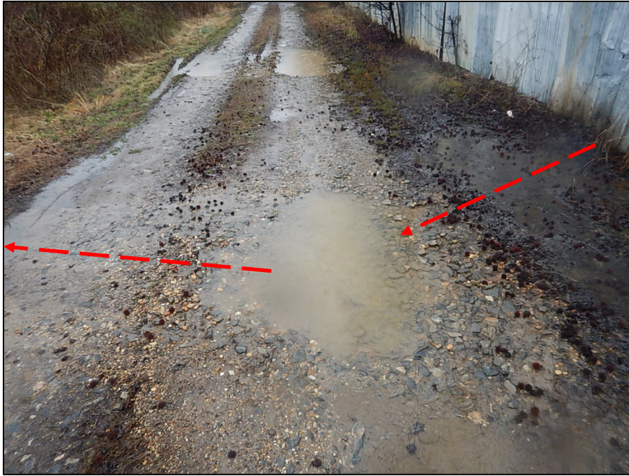
DSCN3946. View, facing northwest, of pooled stormwater that was observed to flow from the Facility downgradient to the southwest offsite location (photograph was taken offsite).
