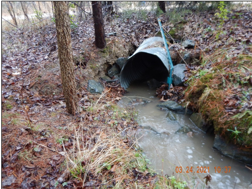
DSCN2175. View, facing north, of flow entering a culvert that collects flow from the drainage ditch and runs under Huntington Lane. Note the flow was turbid.
