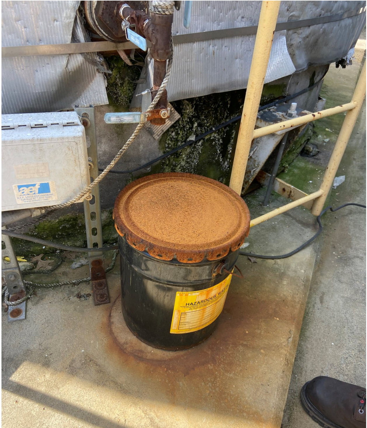
Figure 7: Corroded 5-gallon satellite hazardous waste drum with improper labeling inside Tank Farm #4.
