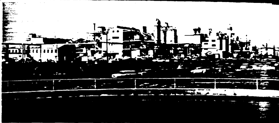
New plant unit at Sayreville, New Jersey for the production of titanium pigments by the chloride process.
