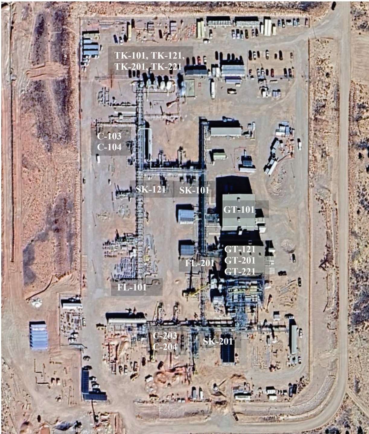
Figure 1: Walker Hollow Compressor Station Aerial View
