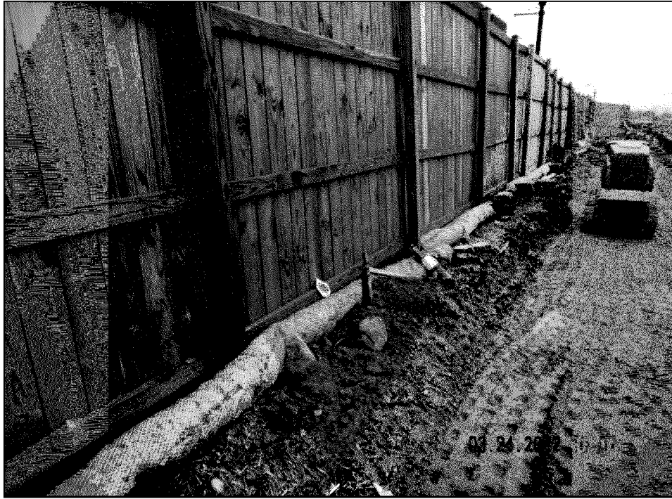
Photograph 25. (DSCN3948.JPG) View, facing northwest, of a filter sock along the west perimeter.
