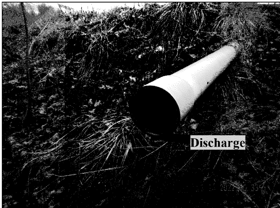
Photograph 76. (DSCN4009.JPG) View of the unlabeled dripping pipe shown in Photograph 75. The EPA Inspection Team did not observe signs of pollutants originating from the discharge, such as sediment, foam, or discoloring.
