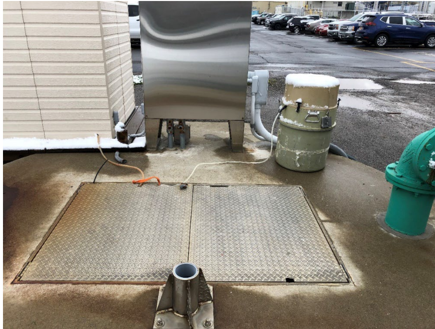
Photo #1. Pretreated effluent from the On-Site Pretreatment System was sampled at Cedar Street Discharge monitoring location (Outfall 001).
