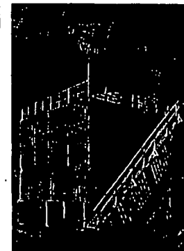
5 Cooling tower, induced-draft fan type, cools water for condensing unit, left
