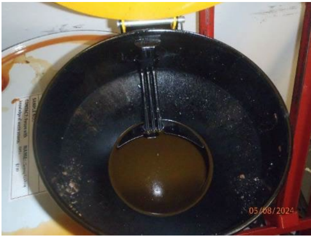
Picture 18 – Storage Room for Used Oil Pads, Drums & Batteries used oil container overfill in funnel
