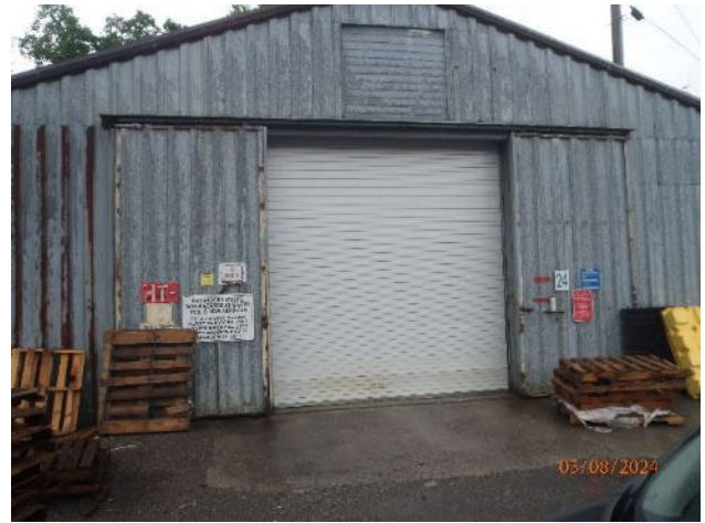
Picture 27 – Hut 24 CAA
