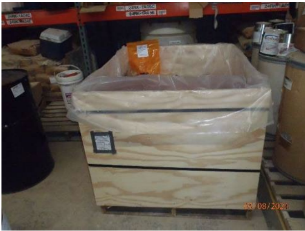
Picture 36 – Hut 24 CAA lead acid batteries
