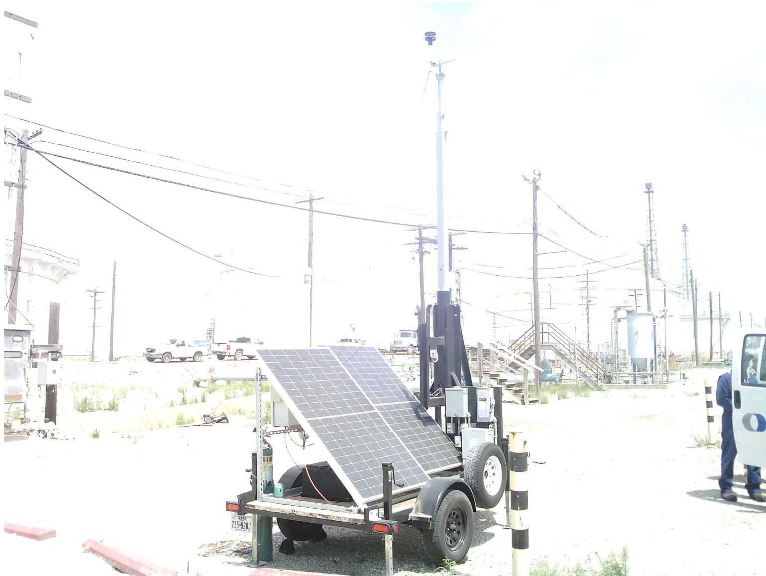
Photo 056: Aecom eGC near tank G-313 - 4/18/2024 14:09 FLIR0056.jpg
