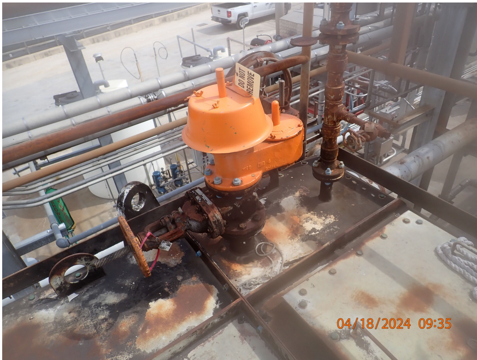
Photo 022: CPI #2 Vacuum Breaker - 4/18/2024 P4180022.jpg
