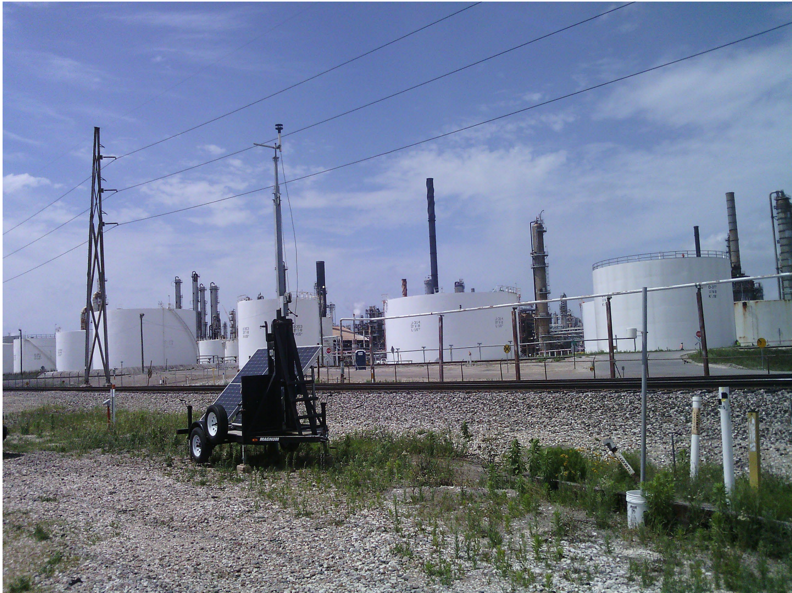
Photo 057: Aecom eGC near Shelter 5 - 4/18/2024 14:29 FLIR0057.jpg
