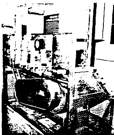
Shown is one part of the breathing air processing station at the Los Angeles City Fire Department—the compressor/purification unit. The compressor prepares the air for purification the removal of all harmful matter.
