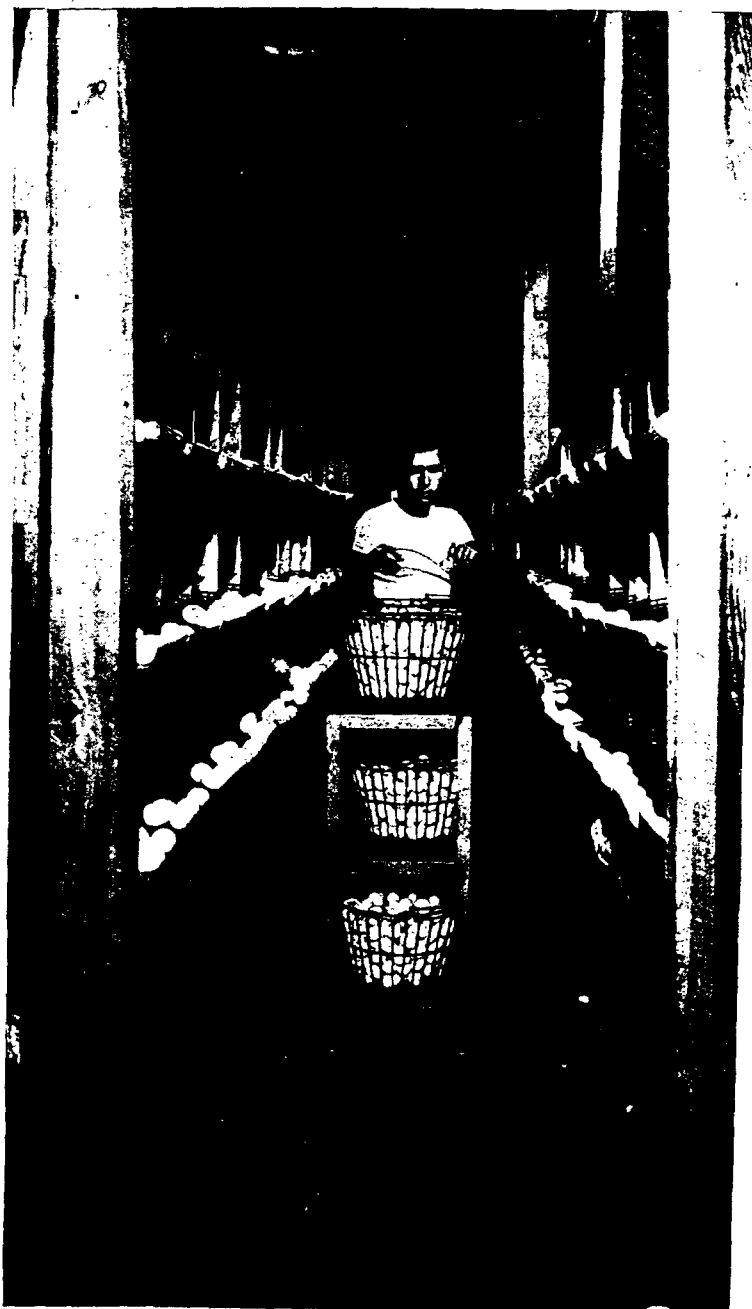
Egg gathering is easy for Marvin Bouse with roll-through aisle nests. Eggs roll toward center aisle, where cart containing three tiers of egg baskets is used to pick them up. Ventilating duct shown above is covered with 25/32-in. asphalt impregnated USG Sheathing.
