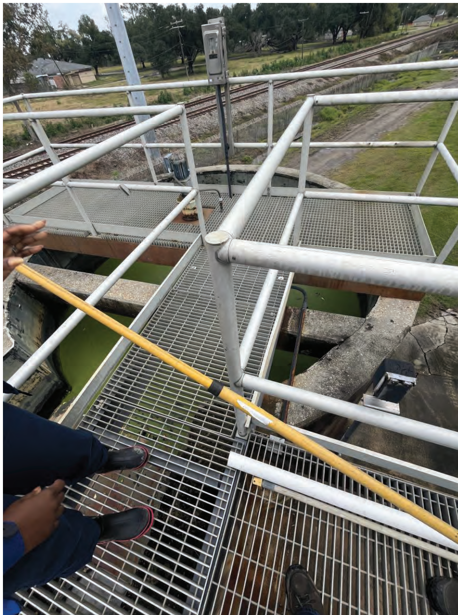
River Road WWTP Out of Service Grit Chamber
