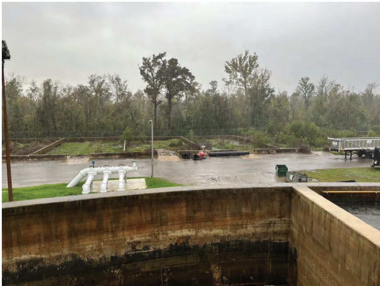
Woodland Treatment Overgrown Drying Beds
