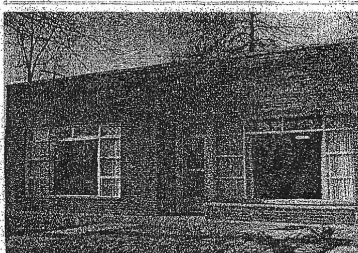
Smart new building shown above is the recently completed home of the DuBois-Webb Company, Fisher agency in Detroit. The building was first occupied by DuBois-Webb personnel last December and with the coming of spring, they wanted the rest of the Fisher-Governor organization to see their new place. The address is 19951 James Couzens Highway, Detroit 85.
