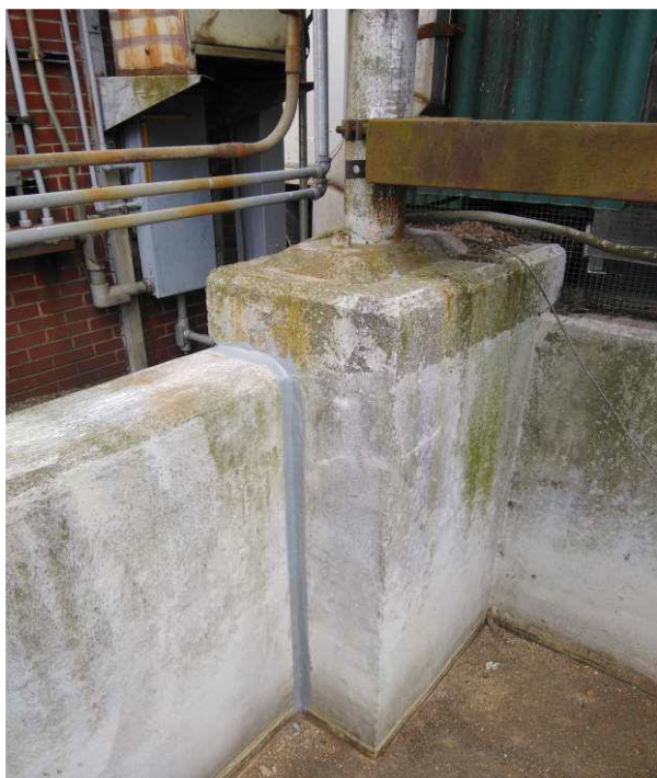
Photo 15: Bldg. 285 HWDU-30. Photograph provided by the facility on May 20, 2021. Repairs have been completed.
