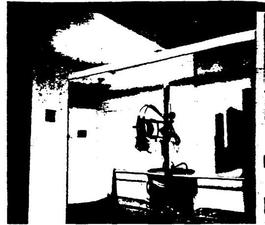
X-Ray room in civilian personnel medical department. Wall panels and screen are of lead covered plywo.
