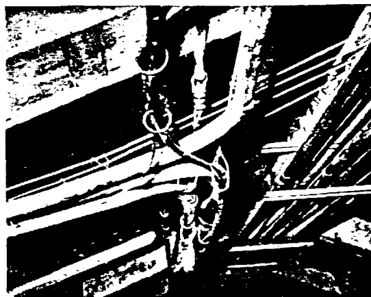
Lead sheathed telephone cables starting here circle the building just under the roof.
