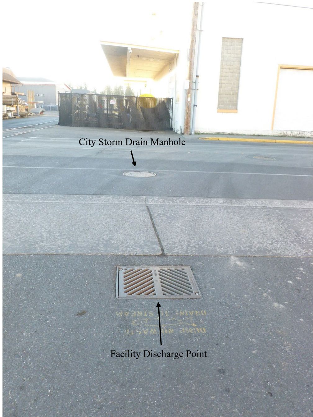
Photo 1 / P1010223 – Discharge Point to City Sewer, facing west
