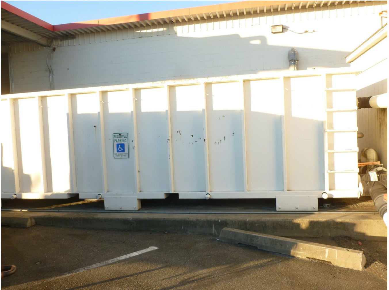
Photo 6 / P1010223 – Discharge Point to City Sewer, facing west
