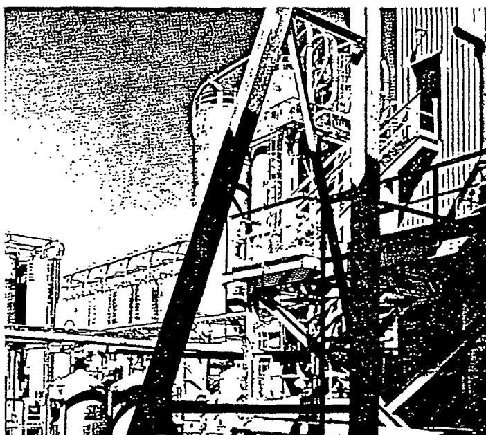
New low-density polyethylene plant in the Texas Division is based on a technologically advanced process for producing resins for high-clarity film.
