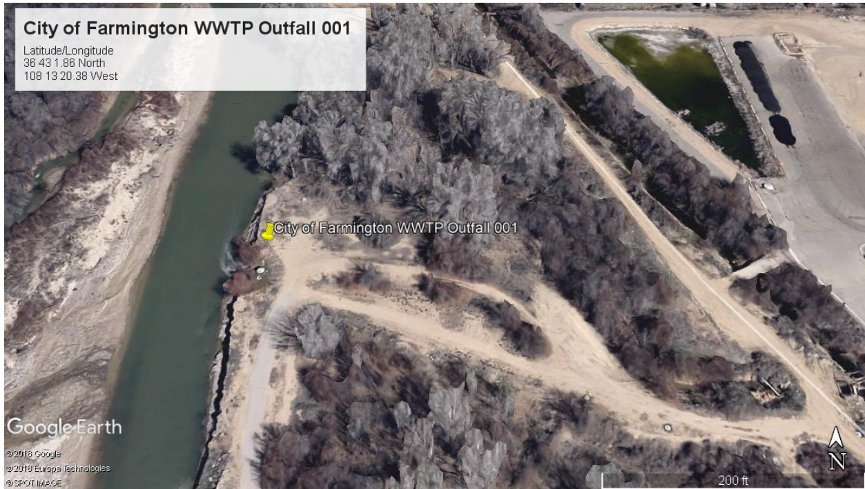
Aerial Image #2: Overall view of the City of Farmington’s Wastewater Treatment Plant outfall 001. Aerial from Google Earth maps.
