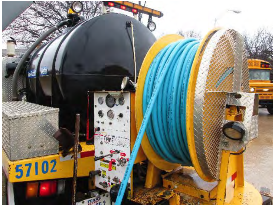
Photograph 34. Jet Truck Crew – View of the jet hose.
