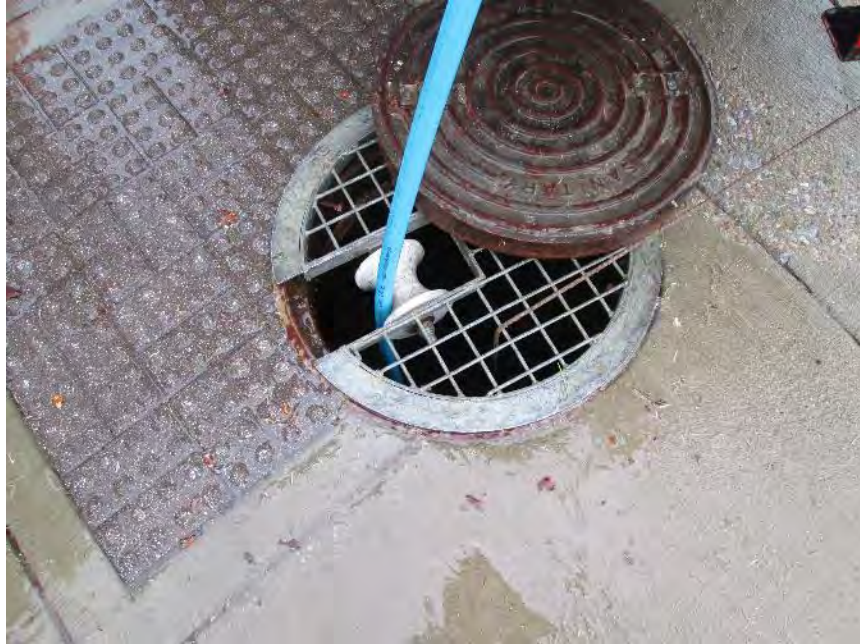
Photograph 33. Jet Truck Crew – View of a fall protection manhole cover used by operators while jet cleaning. The manhole was positioned on the edge of a sidewalk ramp.
