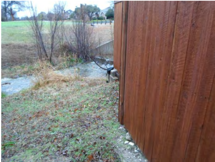
Photograph 48. Lookout Lift Station – The station was located within 20 feet of a small stream.
