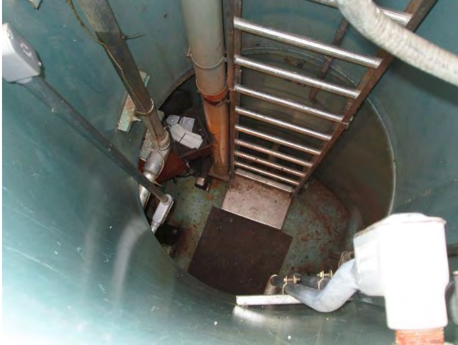
Photograph 13. Meredith Lift Station – View inside the station's dry well.
