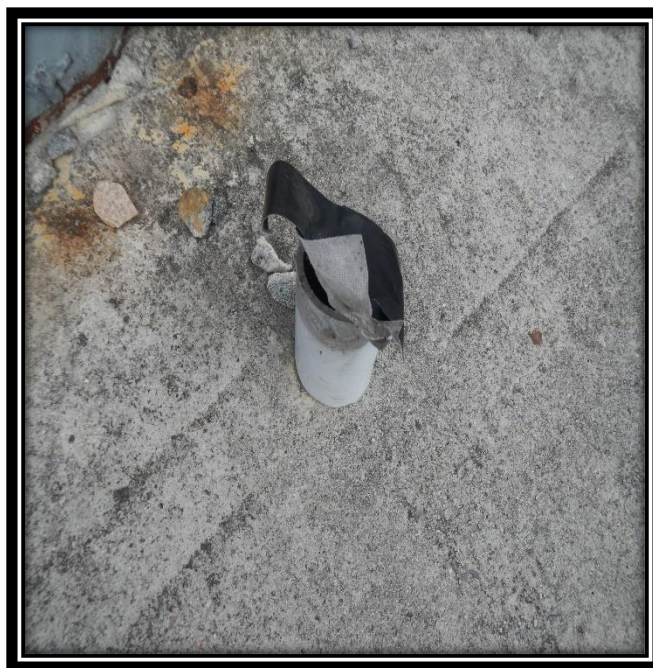
Image 2 Opening in the well pad
