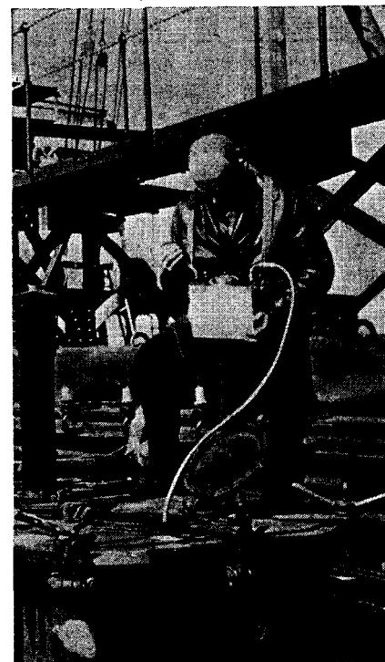
Figure 10. Testing with a combustible gas indicator aboard a tanker. See paragraphs 51 to 53.)
