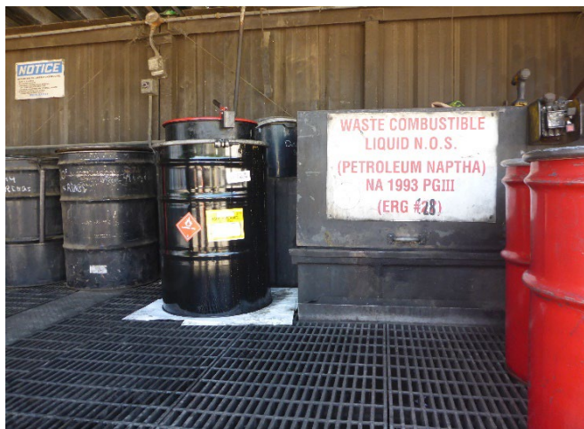
Photo 4: One 55-gallon container for accumulating hazardous waste branch debris in the Return and Fill SAA.
