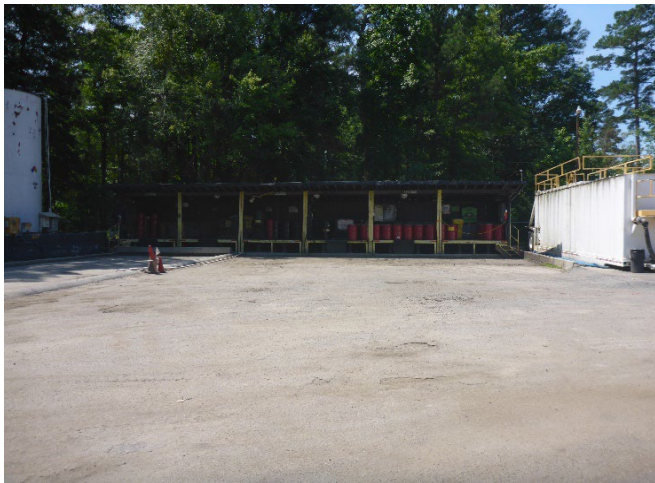
Photo 3: Return and Fill Station.
