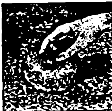
Through the use of the stipple sponge old worn floors may be given a smart, decorative pattern.
