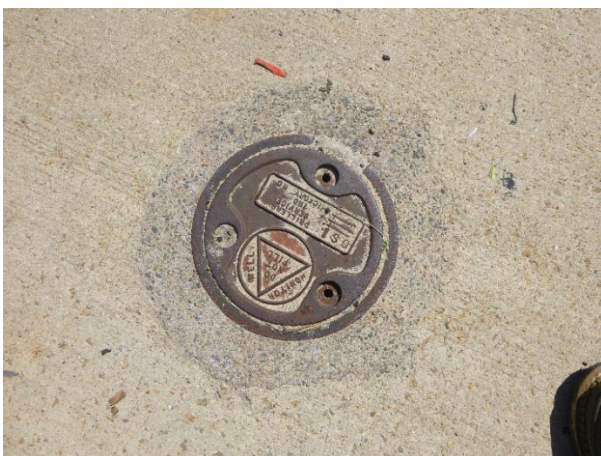
Photograph 56: Monitoring Well.
