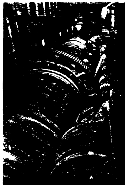
Rotary kiln being installed in first Canadian titanium pigment plant, under construction by a Company subsidiary.
