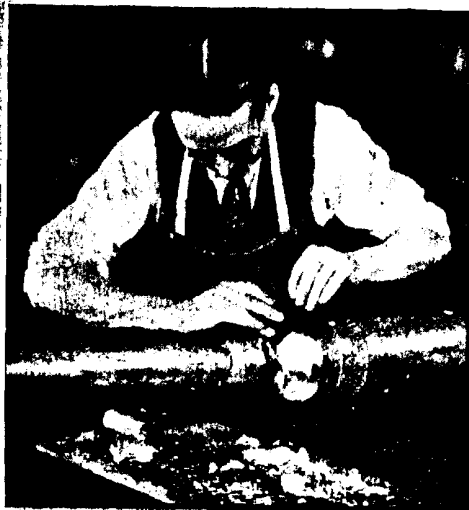
Wiping a soldered joint on a lead-covered telephone cable.
