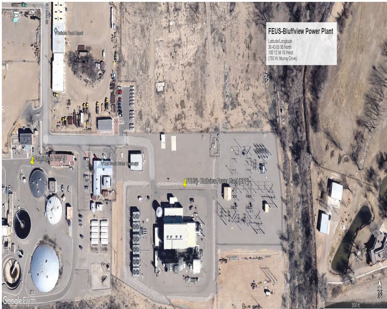
Aerial Image #1: Overall view of the FEUS-Bluffview Power Plant. Aerial from Google Earth maps.
