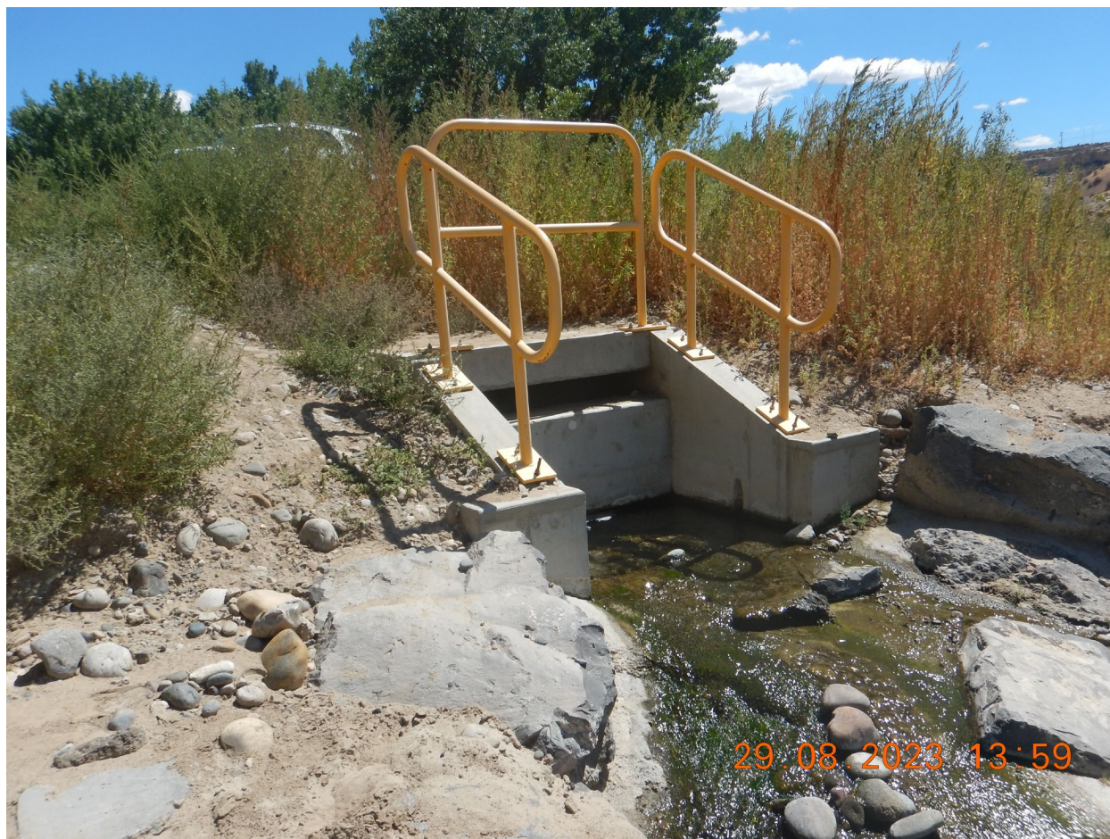
View of the FEUS-Bluffview Outfall discharge into the Animas River. (DSCN2634). Photographed by D. Esparza
