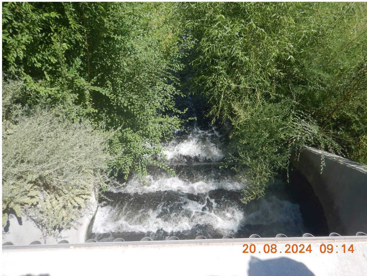
View of Outfall 001 downgradient toward the Rio Grande. (DSCN2716) Photographed by E. Yurk
