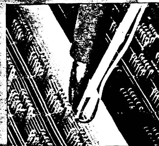
Soldering a strap wire on a crossbar switch in a telephone installation.
