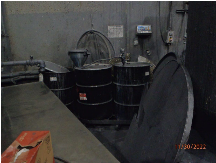
Figure 8: PB300016.JPG – Solvent Feed to Solvent Recovery Still
