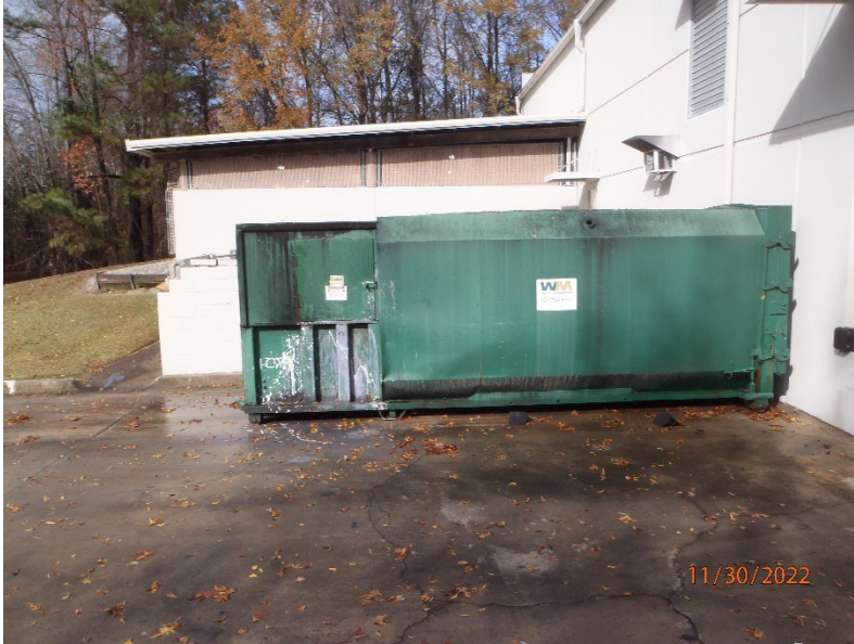
Figure 15 – PB300030.JPG – Solid Waste Dumpster
