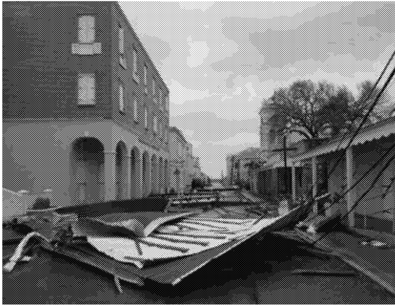
Debris blocking streets in San Juan, Puerto Rico (Photo courtesy of U.S. EPA, September 26, 2017)
