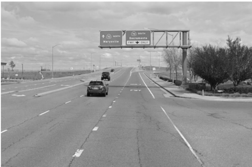
Figure 4: Existing Plumas Lake Boulevard Interchange (Phase 1)
