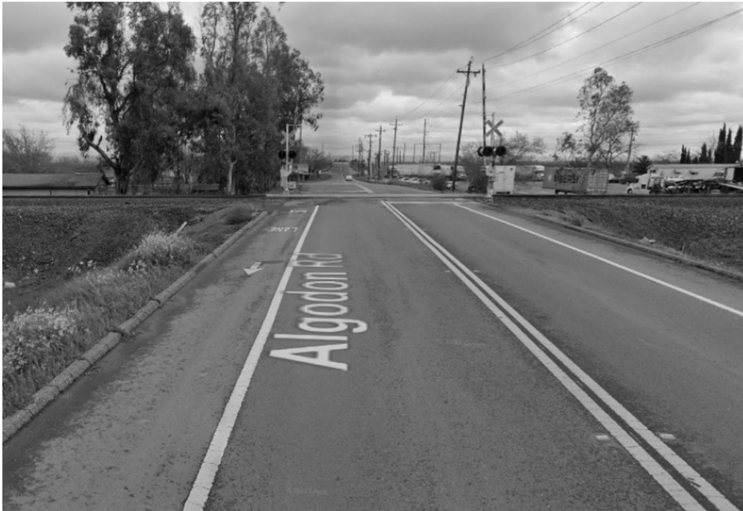
Figure 3: Existing Union Pacific Railroad Crossing at Algodon Road
