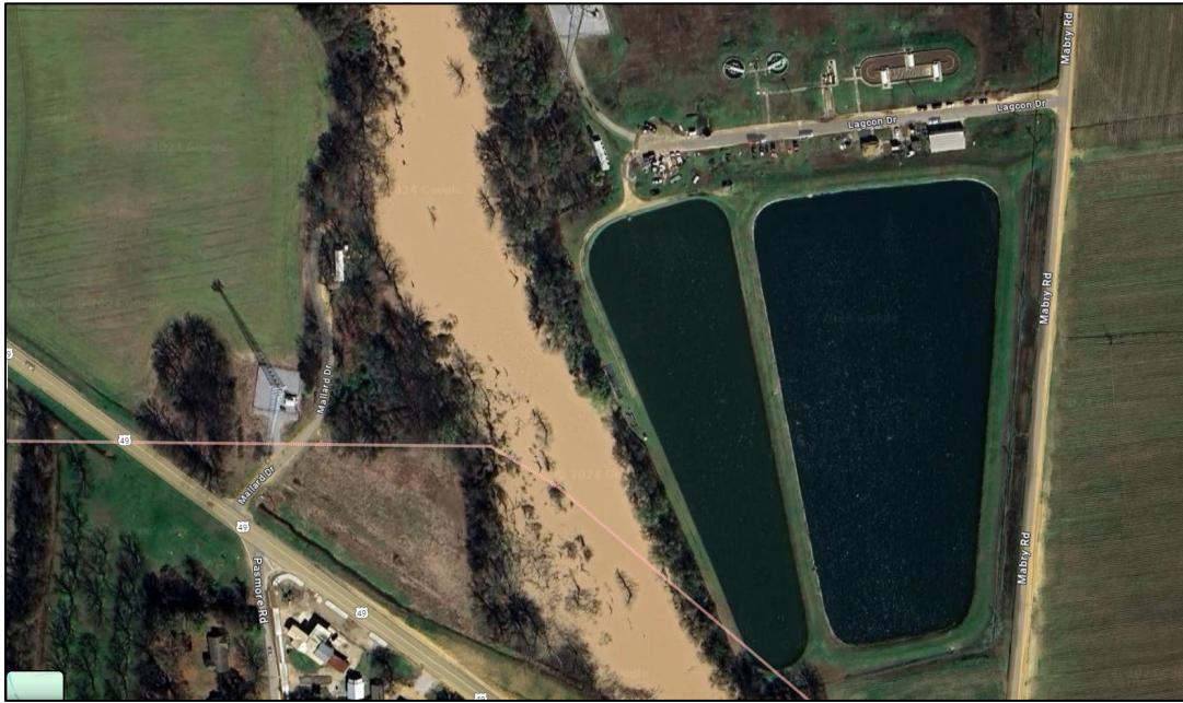
Figure 1. Aerial View of Facility (Oxidation ditch and secondary clarifiers to the north; lagoons to the south). Hopson Bayou to the west.
