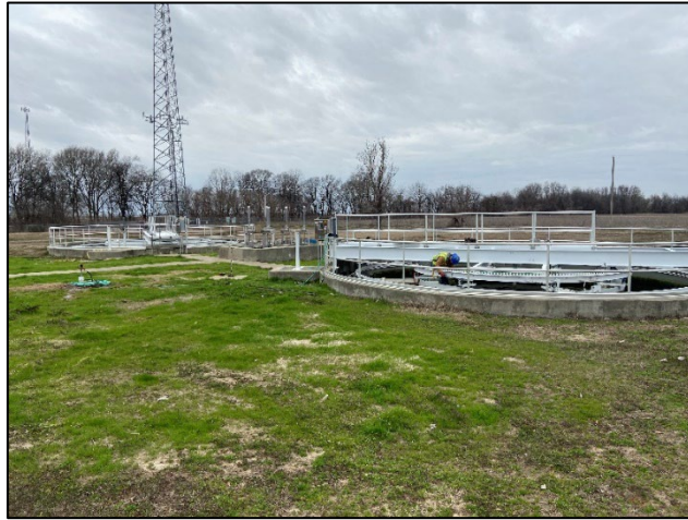
Photo 4: Clarifiers (clarifier on right out of service).
