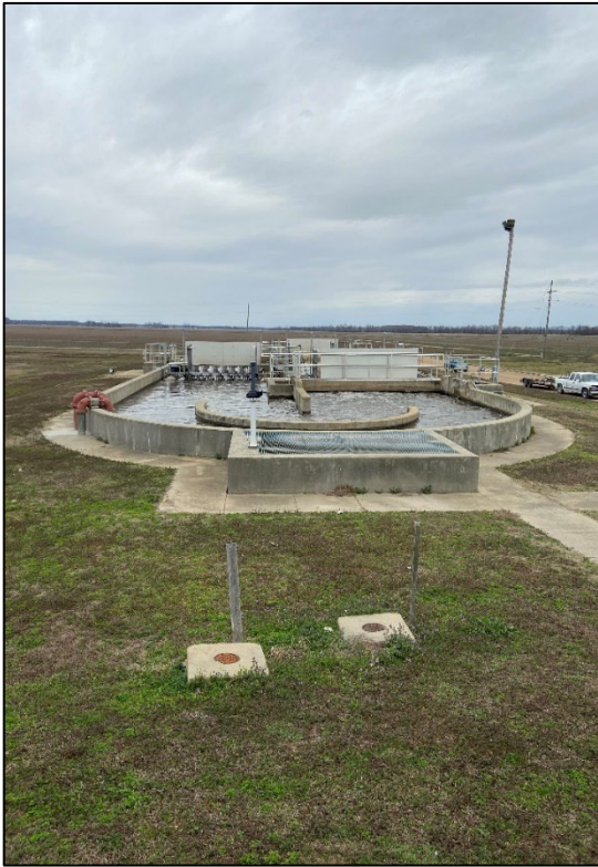
Photo 3: Oxidation ditch.
