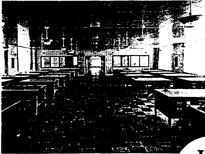
Acoustic Ceiling in the Bridgeton, N. J. Offices of Owens-Illinois Glass Company.
