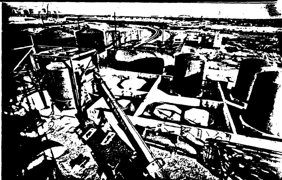
Bulk storage construction for expanded blending facilities at Edwin Cooper's Sauget plant began in 1975. The St. Louis, Mo., arch shows in the upper left of the picture.
