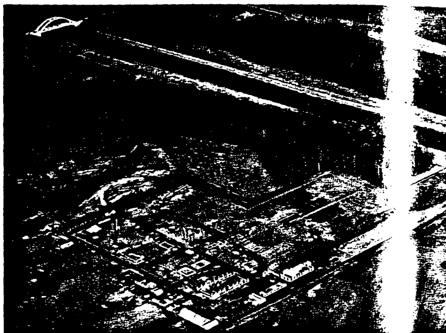
Construction began in September 1975 on an aluminum alkyls plant in Feluy, Belgium. The plant, located on the Charleroi-Brussels canal, is scheduled to open in mid-1976.
