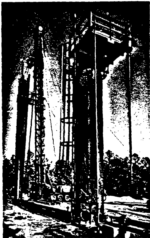
A brine well is serviced as part of drilling operations at Magnolia, Ark.
