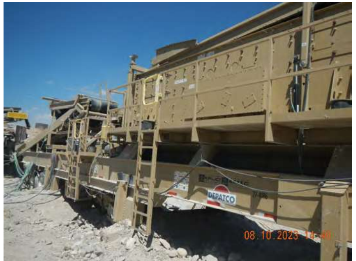
Photo #:20 (DSCN3404) Description: Photo of the crushing operation.
