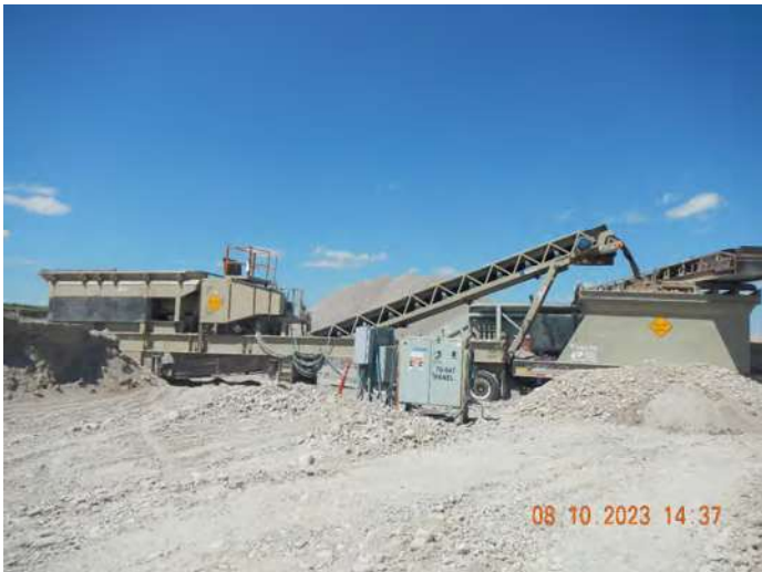
Photo #:19 (DSCN3403) Description: Photo of the crushing operation.
