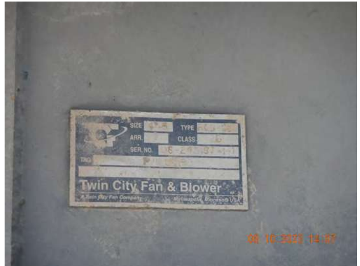
Photo #:02 (DSCN3386) Description: Twin City Fan & Blower nameplate associated with the hot mix asphalt plant, currently staged and not operating.
