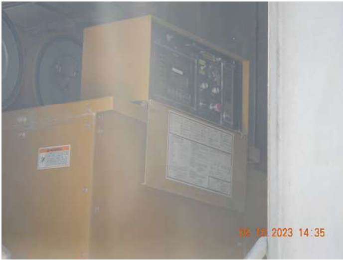
Photo #:17 (DSCN3401) Description: Photo of the display of the Caterpillar model 3512 (EU ID: Gen01)
