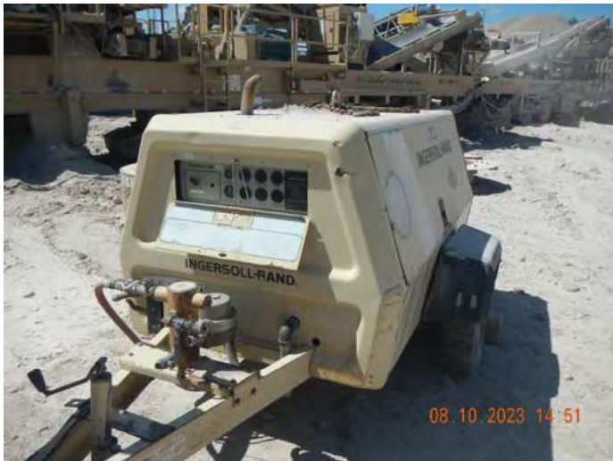
Photo #:23 (DSCN3409) Description: Photo of an auxiliary generator near the crushing operation. Ingersoll-Rand.
