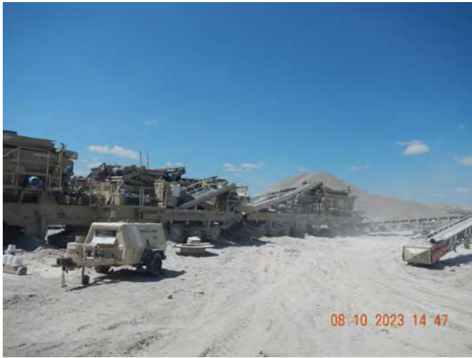
Photo #:21 (DSCN3405) Description: Photo of the crushing operation
