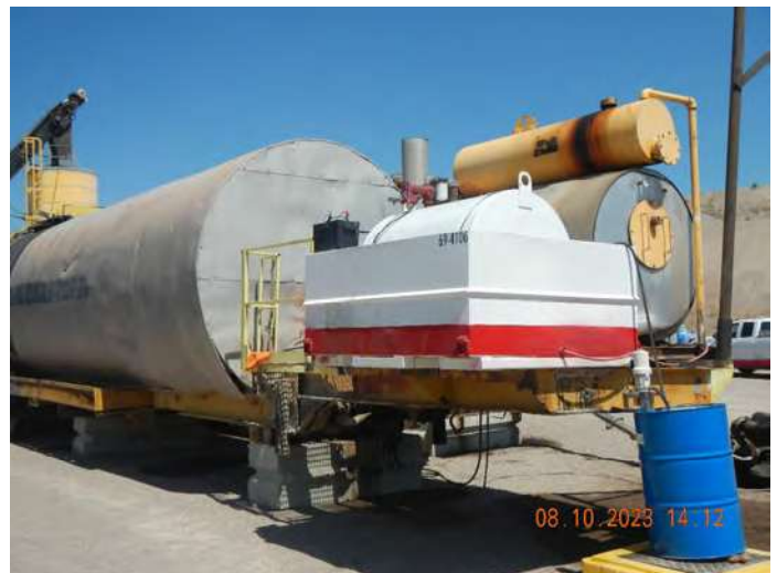
Photo #:04 (DSCN3388) Description: Photo of auxiliary heater and asphalt oil storage tanks at the hot mix asphalt plant.
