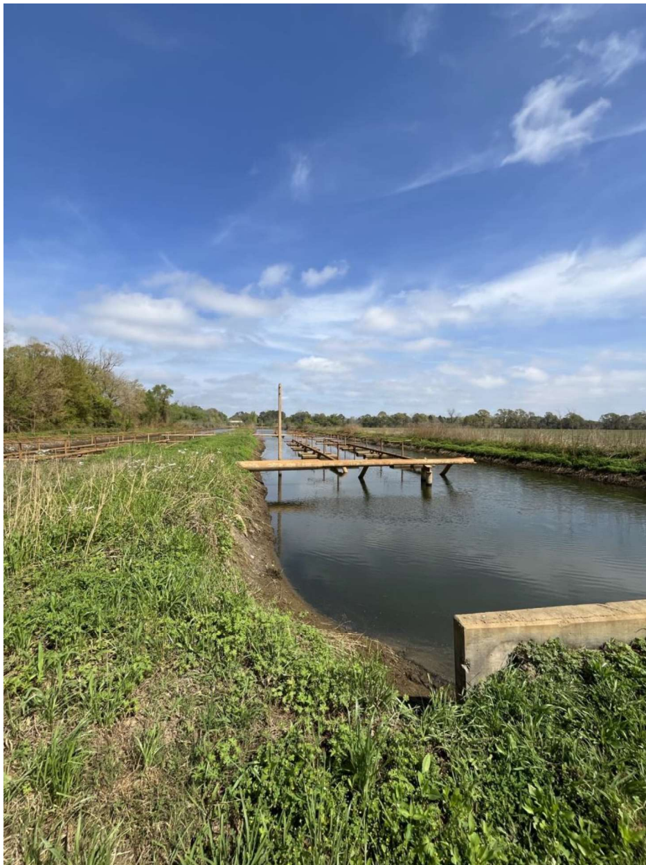
West Aeration Basin
