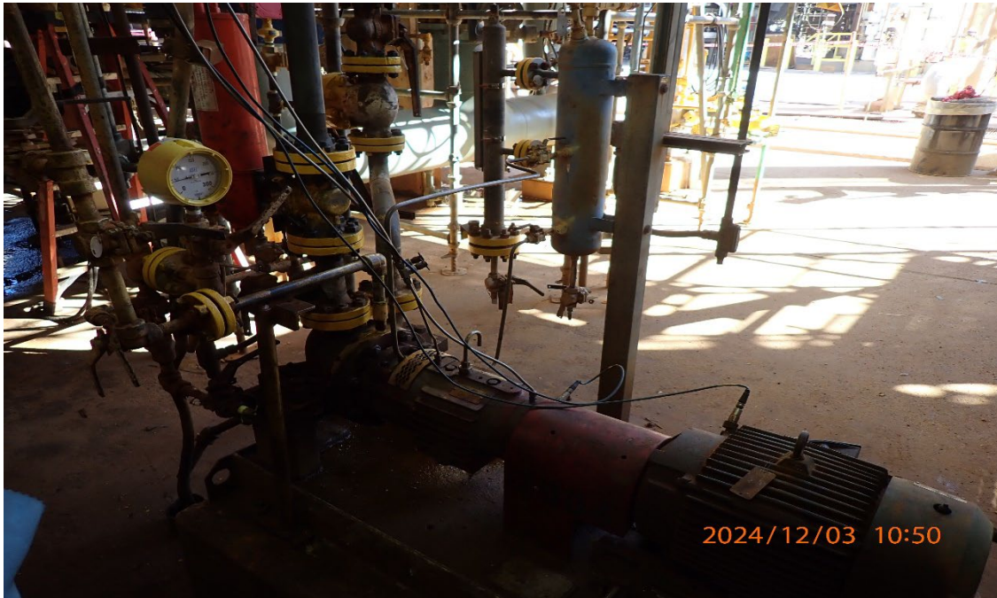
Photograph 27 - File: PC030040.JPG Acid rerun pump in the Alky Unit.
