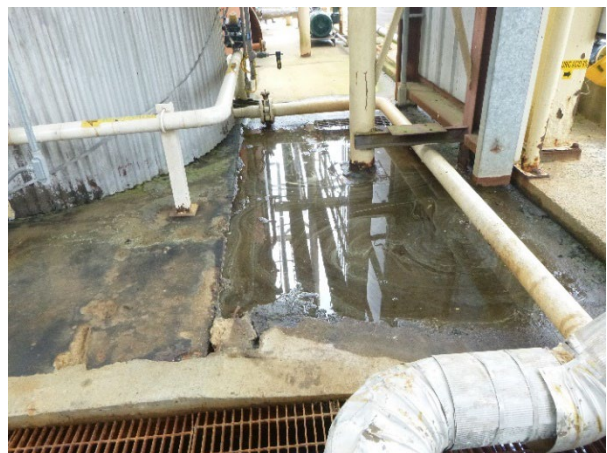
Photograph 21: Hazardous Waste Tank CAA.
