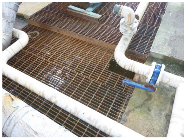
Photograph 20: Hazardous Waste Tank CAA.
