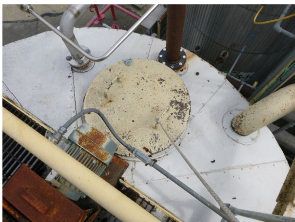
Photograph 24: Hazardous Waste Tank CAA.
