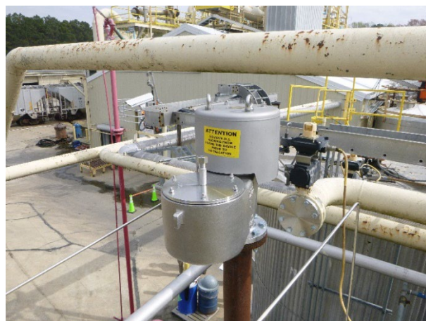
Photograph 26: Hazardous Waste Tank CAA.
