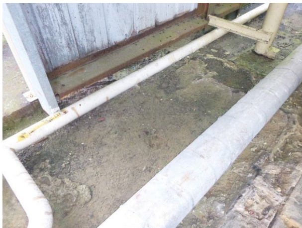
Photograph 19: Hazardous Waste Tank CAA.
