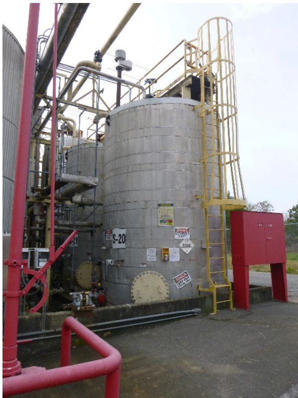
Photograph 18 Hazardous Waste Tank CAA.
