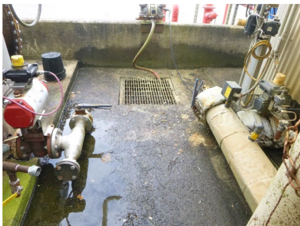
Photograph 23: Hazardous Waste Tank CAA.
