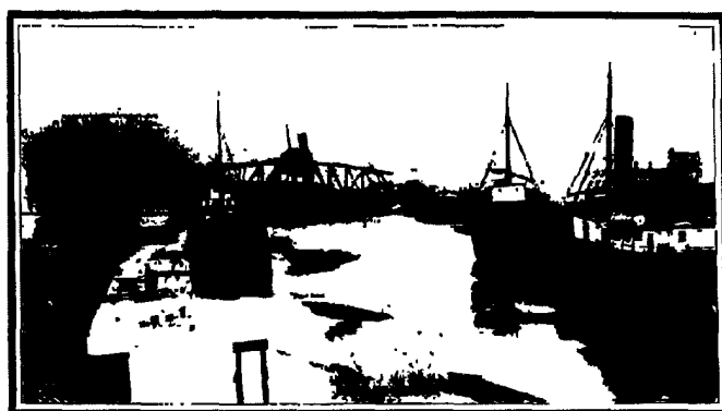
The flooded river looking up stream from the Roof of our factory
