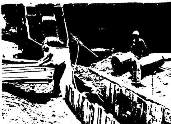
Large diameter, long length clay sewer pipe in fully sheeted trench.
