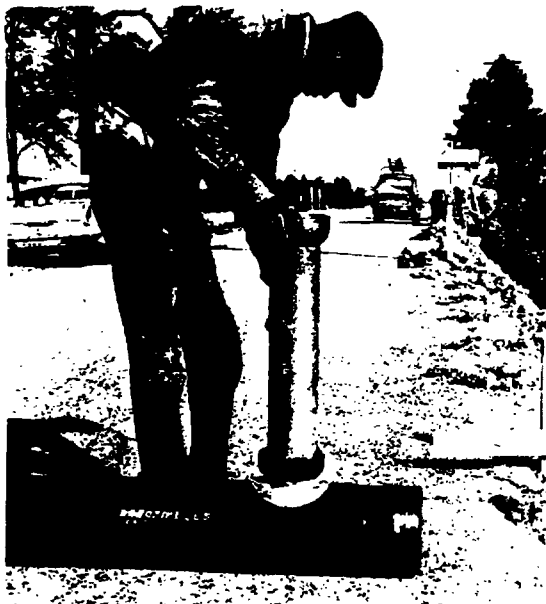
House sewer connection being set into 12-in. bituminized-fiber sewer pipe.
