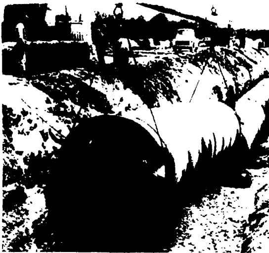
Steel pipeline (96-in.) carries effluent from Baltimore activated sludge plant 4-1/2 in. to steel plant for use as cooling water.
