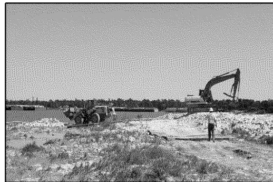
San Jacinto Pits: The potentially responsible party continues with cap repairs on western cell and central berm.
