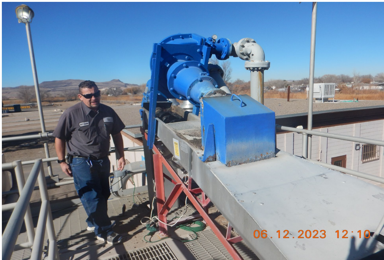
View of the CAS grit chamber screen. (DSCN2649). Photographed by D. Esparza
