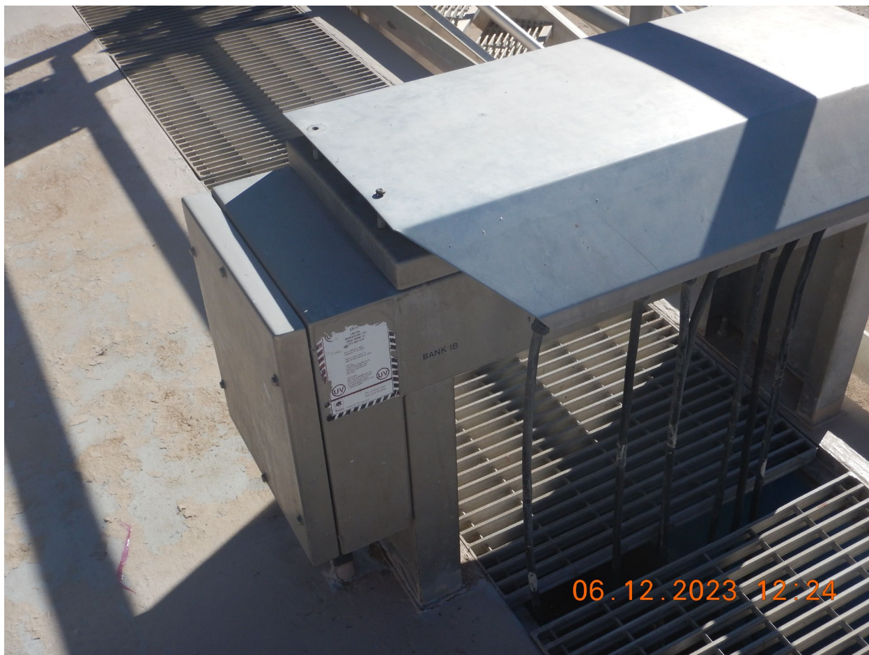
View of the CAS westside Ultraviolet disinfection module. (DSCN2653). Photographed by D. Esparza
