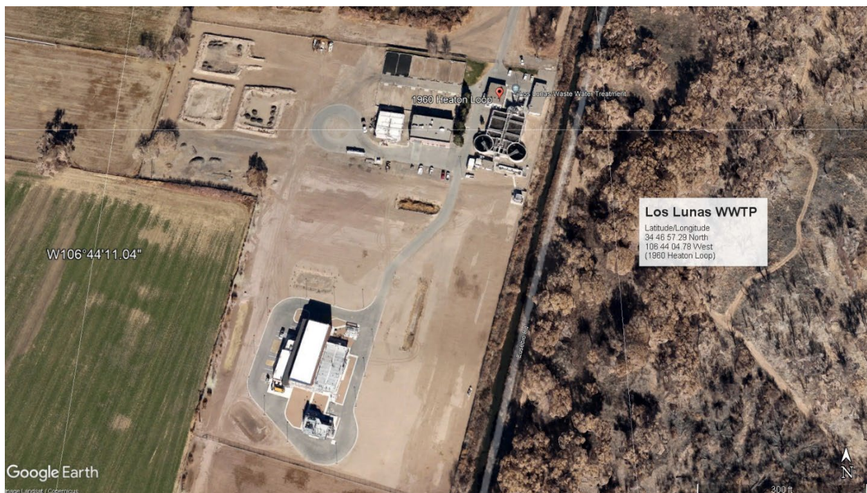
Aerial Image #1: Overall view of the Village of Los Lunas Wastewater Treatment Plant. Aerial from Google Earth maps.
