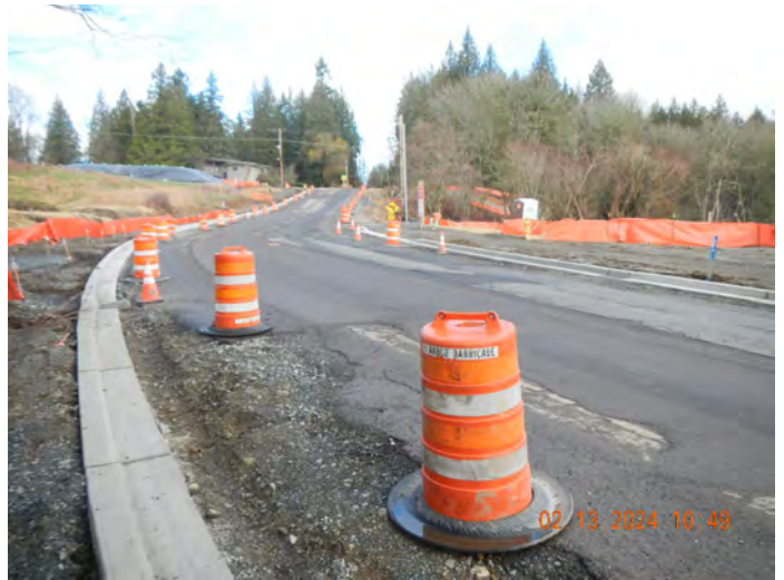
Photo #:12 (DSCN3584) Description: Facing north along Williams Road, photo of frontage area and two roadside catch basins (background) designed to discharge to the roadside ditch south of Williams Road.
