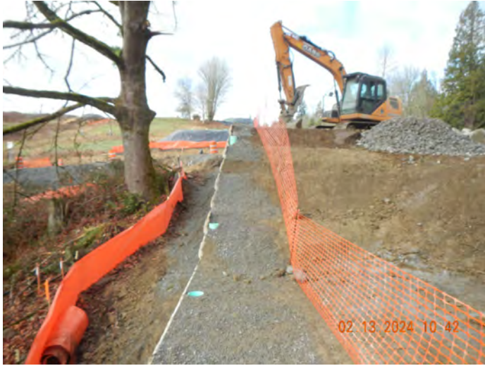
Photo #:09 (DSCN3581) Description: Facing west at “Lot 50” (Lot 52 on map). Area was prepped/work the day prior to the inspection.
