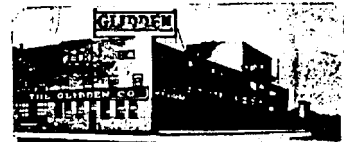
Paint Manufacturing Plant—San Francisco, Cal.
