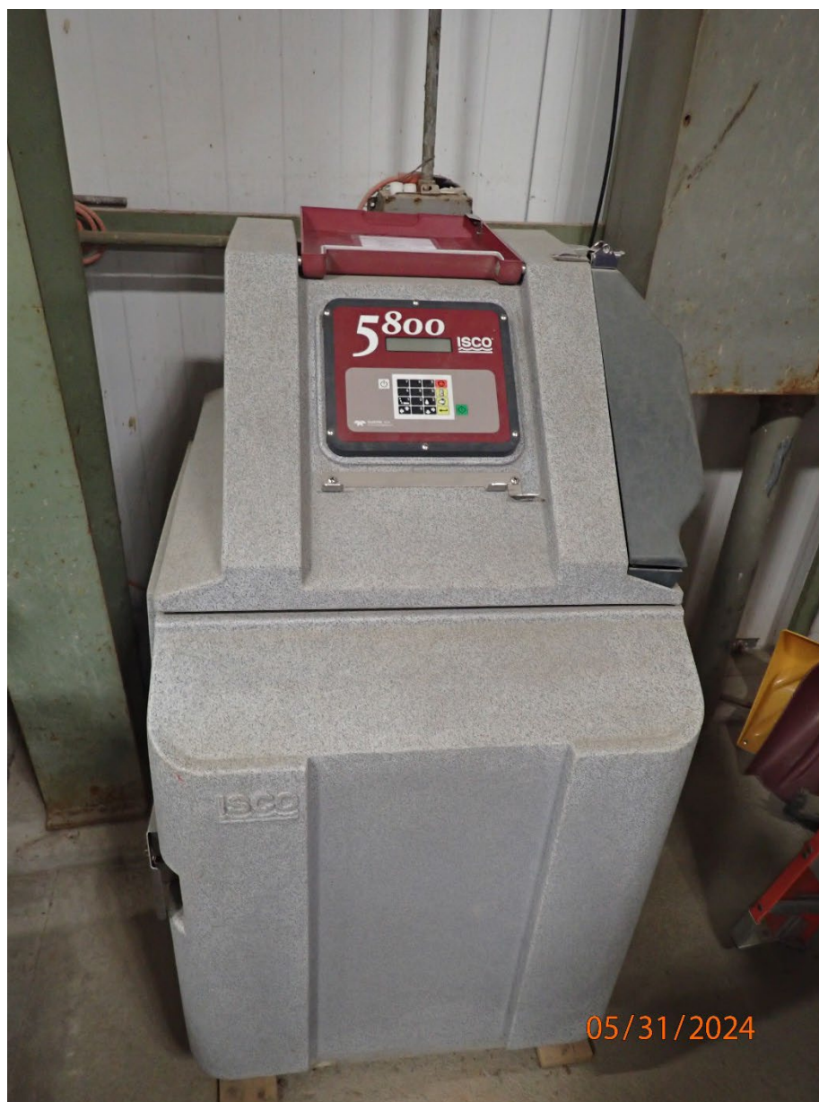
Photo 2- Influent composite sampler
